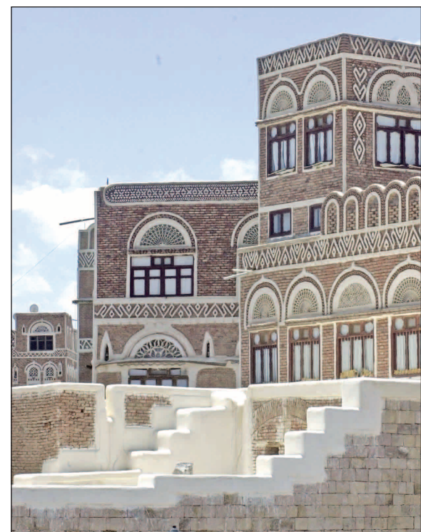
Sana'a architecture runs from rather crude buildings from the 16th century to incredibly detailed 19th century buildings, such as this mansion with intricate, arched fans over windows. The fans are mostly hollow and allow air to circulate.
