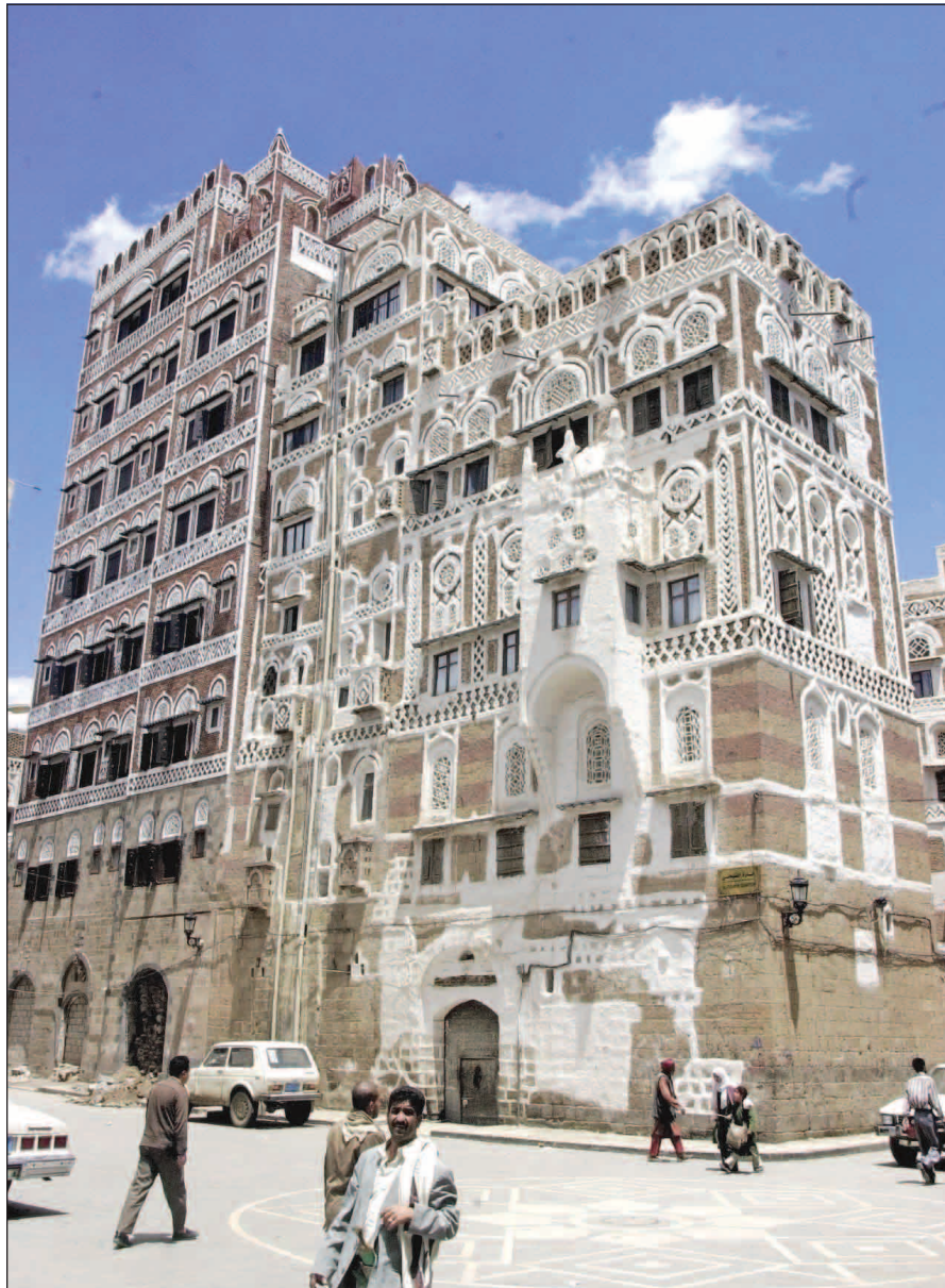
Could buildings such as these in Yemen's old city be the world's first skyscrapers? Some of the multi-story residences are 400 years old, predating Manhattan's high-rise apartments by three centuries.
