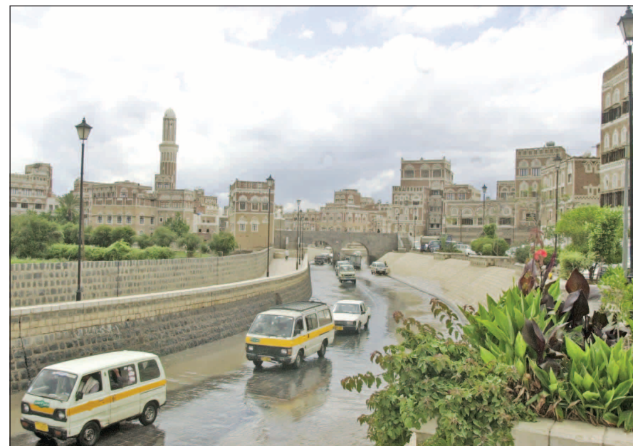
Motorists in Sana'a drive on what was designed as a huge canal, meant to channel storm waters out of the city. When the rains come, heedless drivers often end up with submerged cars.
